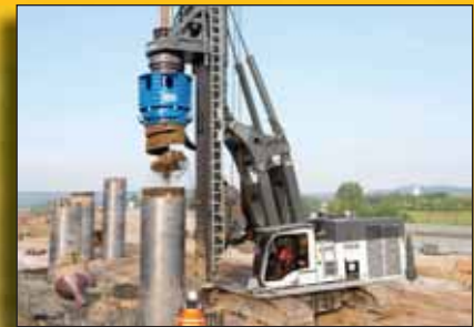
FOUNDATION DRILLING
