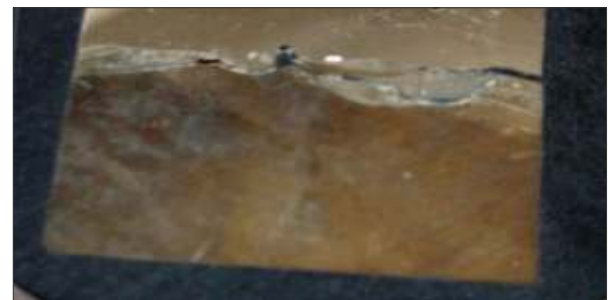
Fig 3 Mounted cross section of the failed frog showing a crack running in the fusion zone of AMS frog and 312 Stainless steel buffer layer.
